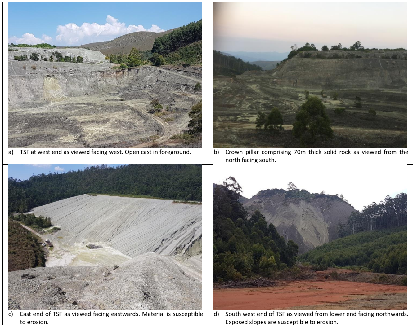
Figure 11 - Selected images of un-rehabilitated Tailings Storage Facility
